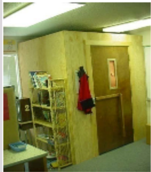
Classroom seclusion room, Kansas
